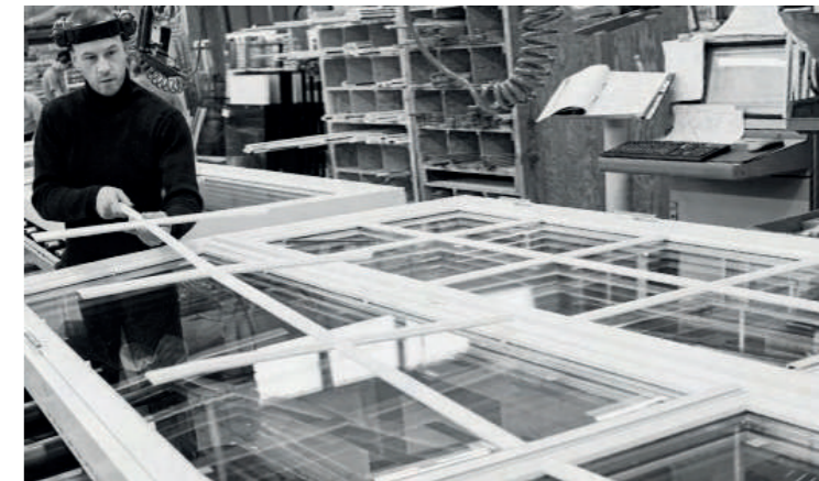
Assembling of plastic windows.
