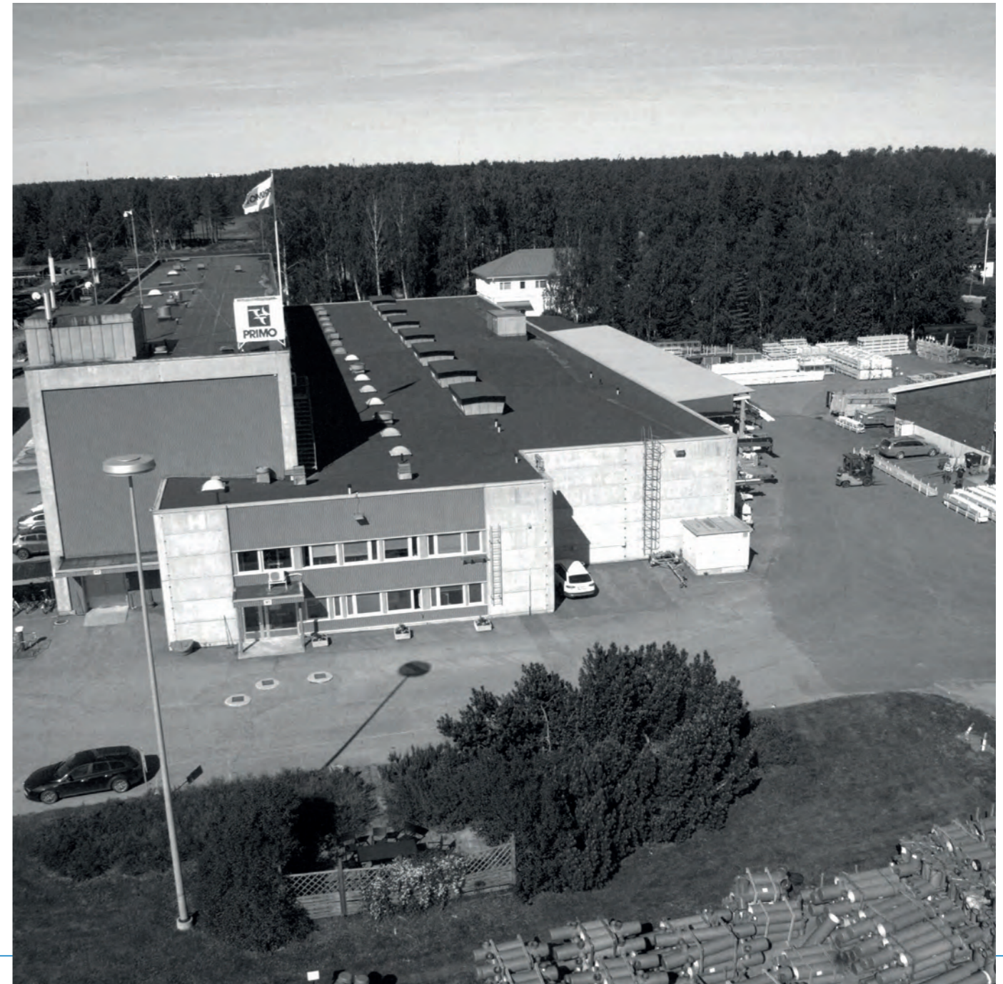
Primo factory in Vaasa, Finland.
